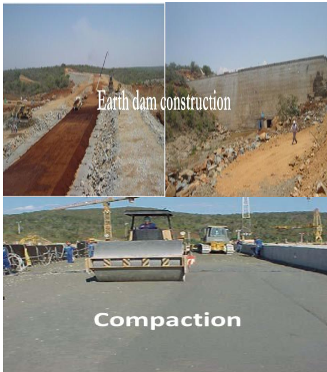
Fig 7. Earth dam construction
